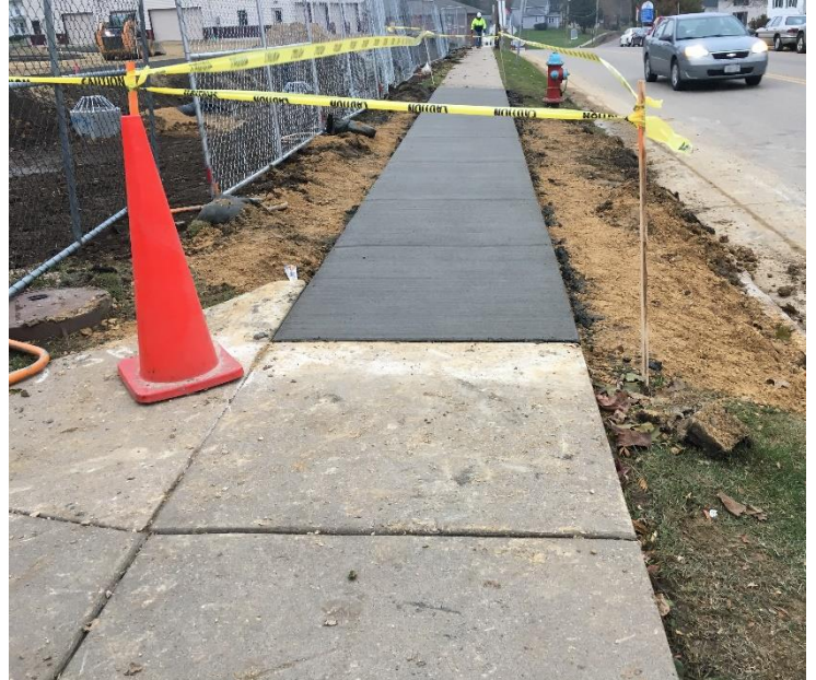
Some new areas of sidewalk were also added near the new Rehab Lot.
