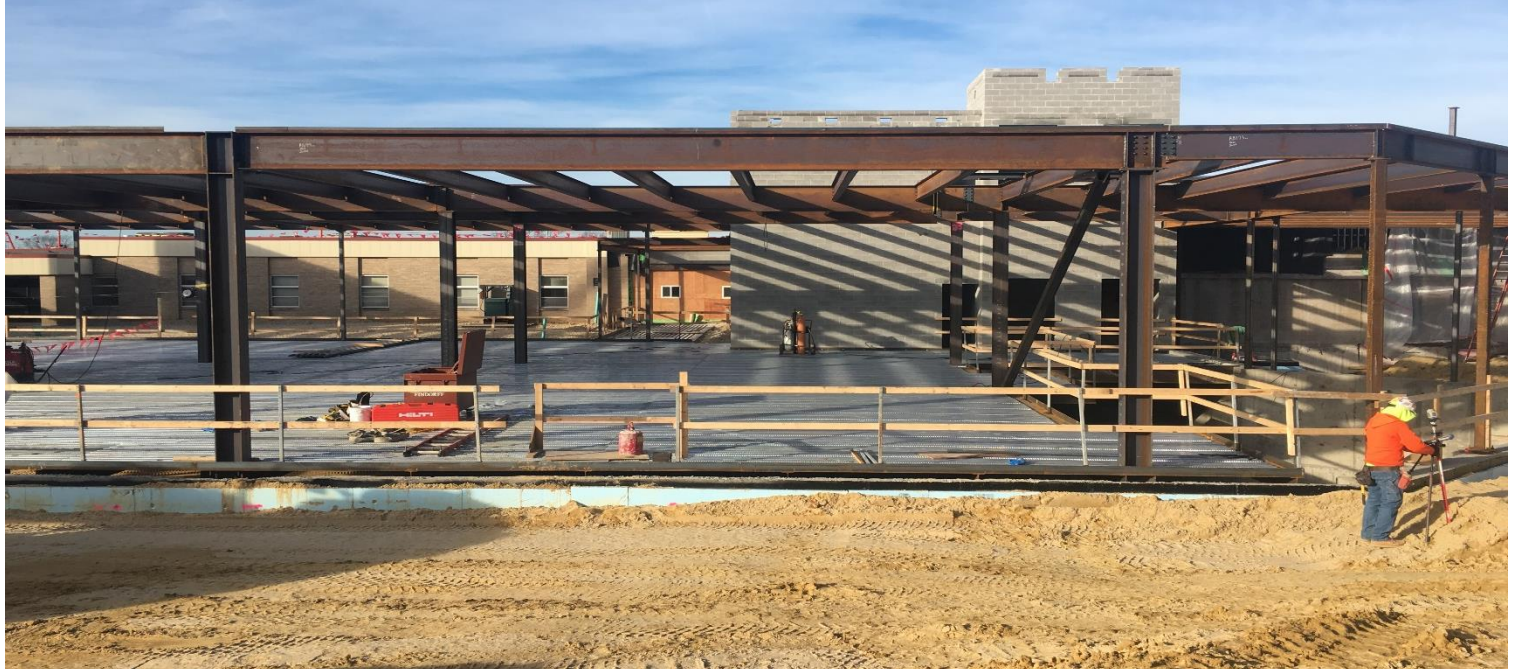
A view of the steel that is in place, along with the decking that will be used to support the concrete floor. To the right you can see one of the team members using surveying equipment to help the crew place their materials in the correct spots!
