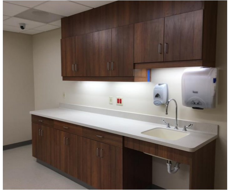
New casework installed in the Pharmacy room. Soon different furniture and shelving will be installed.
