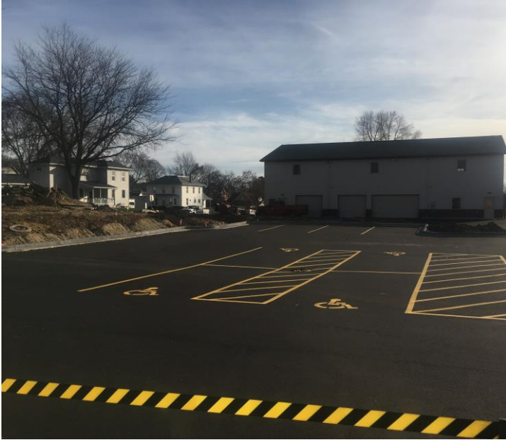
The new Rehab lot is paved and open for business! This can be accessed from the south side of GRHC, just before the construction site.
