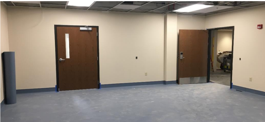
Doors and flooring have been installed in the temporary sterile storage area. This area will be turned over with the Emergency Department.
