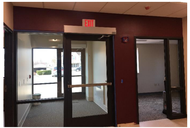
Final coats of paint are being added in the Education Area to complete the space.
